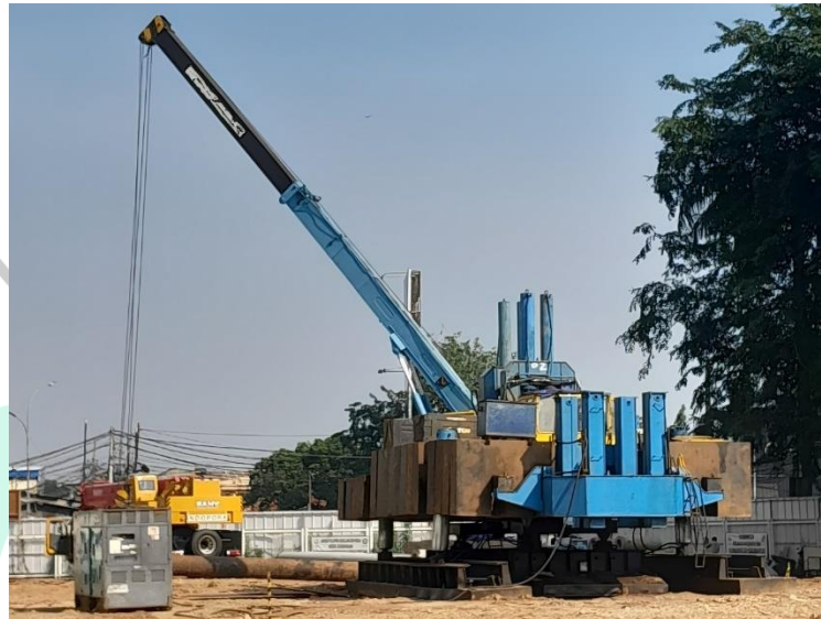
Gambar 3. 13 Hidrolik Statik Pile Driver
