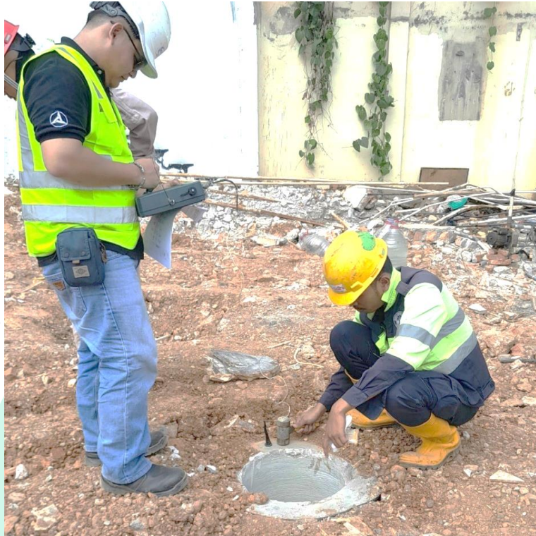
Gambar 3. 35 Pile Integrity Test
