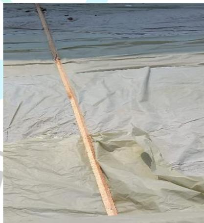
**Gambar 3. 23 Crack Inducer**
