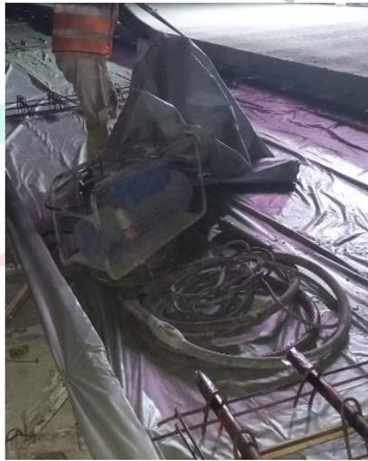
**Gambar 3. 12** *Beton Vibrator*
