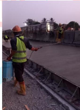
**Gambar 3. 35** Tahapan Pekerjaan *Curing Compound*
