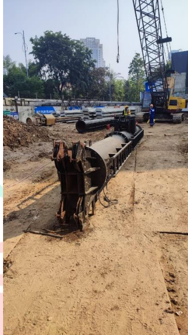
Gambar 3.11 Setting Alat Pancang
