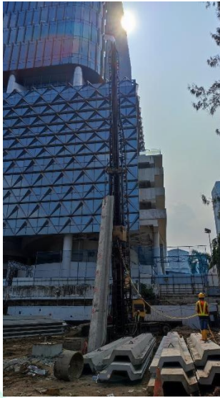
Gambar 3.12 Proses Persiapan Penegakkan CCSP
