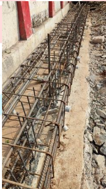
Gambar 3.24 Proses Pembesian Capping Beam
