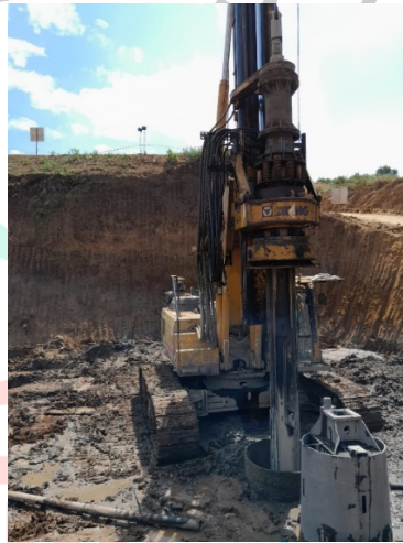
Gambar 3. 24 Hydraulic Rotary Drilling Rig (Sumber : Dokumentasi Pribadi)
