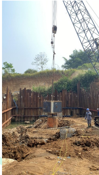
Gambar 3. 35 Pengujian Pile Driving Analysis (Sumber : Dokumentasi Pribadi)
