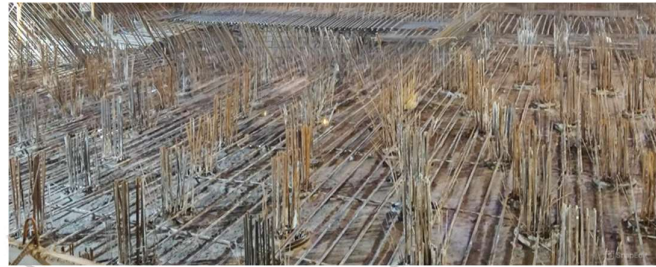
Gambar 3. 41 Pembesian Pile Raft Foundation
