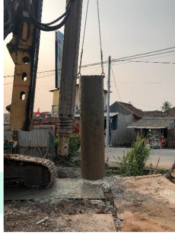
Gambar 3.11 Proses Pemasangan Temporary Casing
