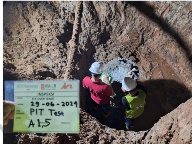
Gambar 3.23 Proses Pengujian PIT Test
