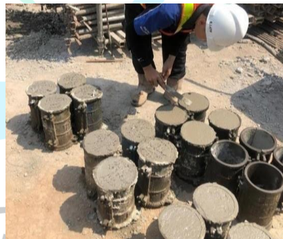
Gambar 3. 21 Beton Ready Mix
