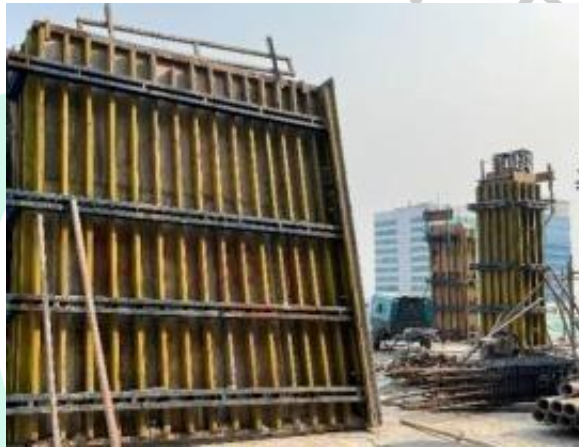
Gambar 3. 77 Perisapan Panel Bekisting
