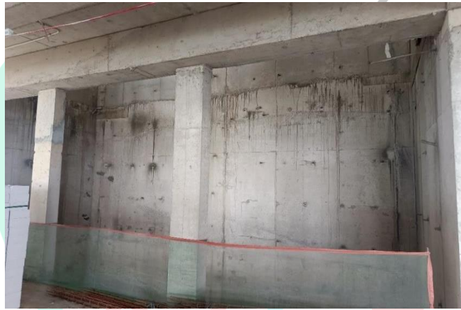
Gambar 3. 67 Core Wall (Dinding Geser)
