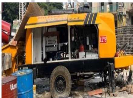
Gambar 3. 19 Concrete Pump Kodok
