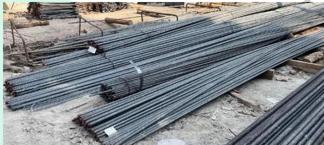
Gambar 3. 22 Stockyard Tulangan Baja
