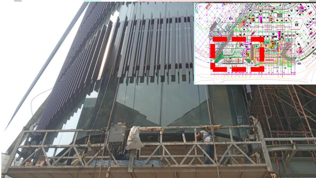
Gambar 3.3 Pemasangan Fasad di Area Mall
