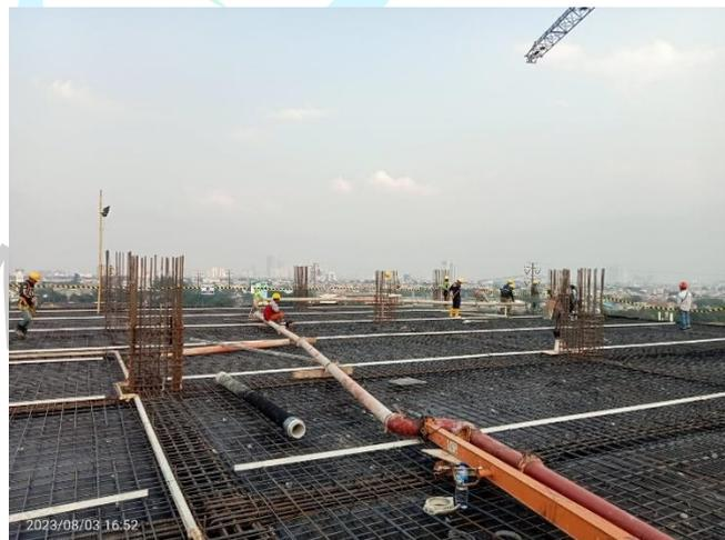
**Gambar 3. 47 Proses Persiapan Pipa Tremie**
