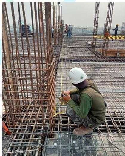
**Gambar 3. 45 Proses Pengecekan Garis Sumbu Balok Dan Pelat**
