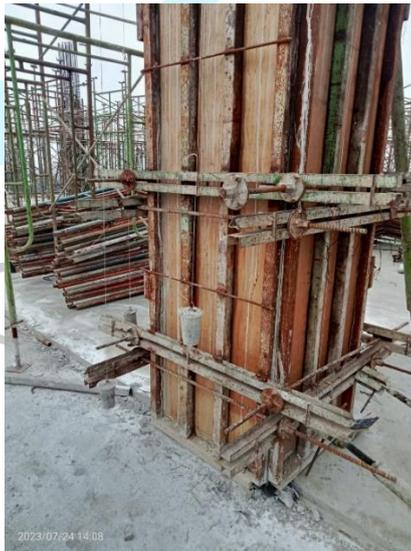
**Gambar 3. 68 Proses Pendiaman Beton Segar Kolom**
