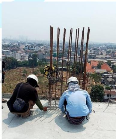
**Gambar 3. 60 Proses Marking As**
