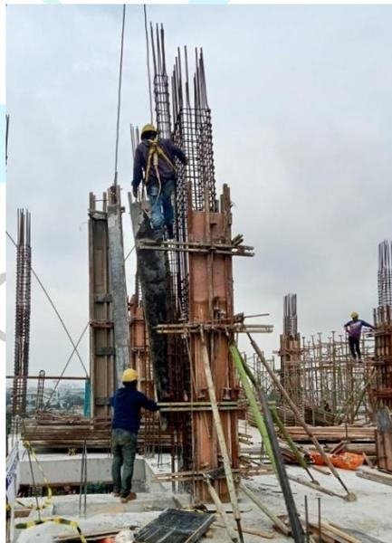
**Gambar 3. 64 Proses Pemasangan Bekisting Kolom**
