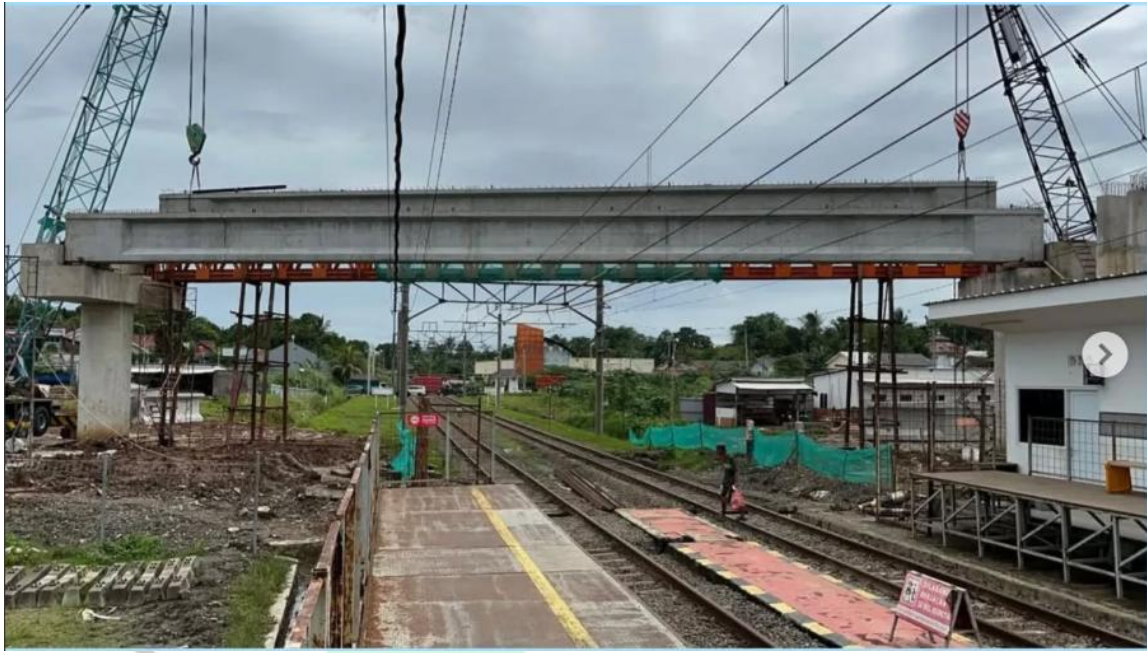
Gambar 4. 2 Pemasangan Girder Flyover Tendjo
