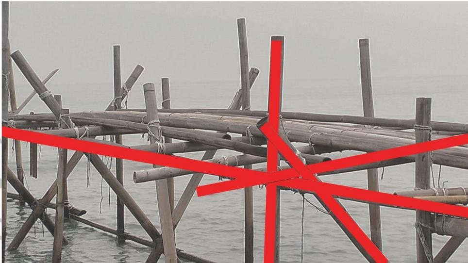
Gambar 2. 18 Stuktur Dermaga Lincak Bambu
