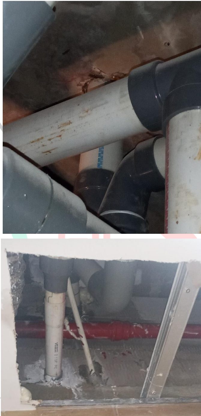
Gambar 3.8 Pengecekan Sumber Kebocoran
