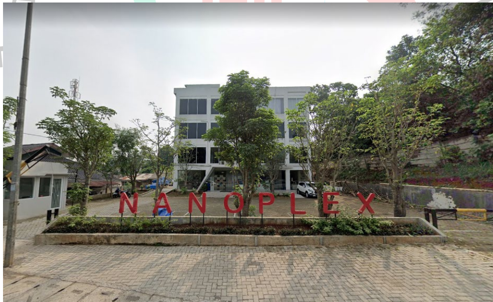
Gambar 1.2. Gedung Kantor PT.Graha Nano Tech Indonesia
