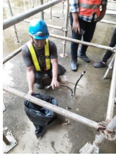
**Gambar 3.45 Proses Menekuk Selang Bagian Outlet**
