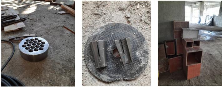
**Gambar 3.12 Anchor Head, Wedges, dan Casting**
