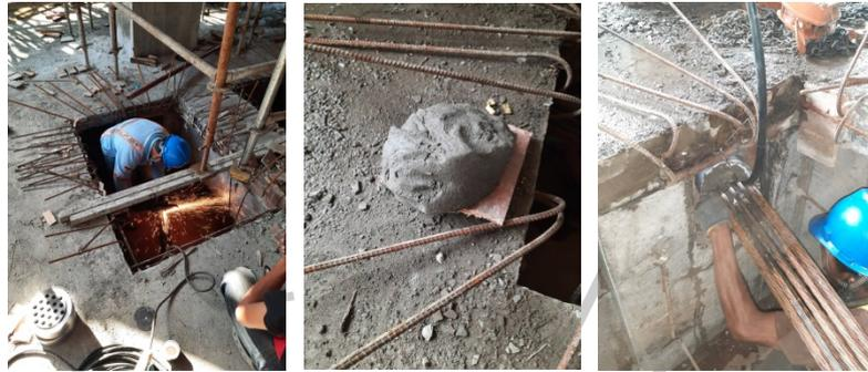
**Gambar 3.42 Proses *Finishing Stressing***
