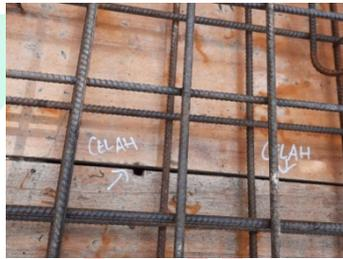
**Gambar 3.5 Pengecekan Papan Bekisting**
