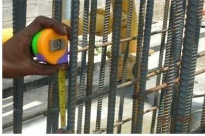
**Gambar 3.21 Proses *Marking* Posisi Ketinggian *Support Bar***
