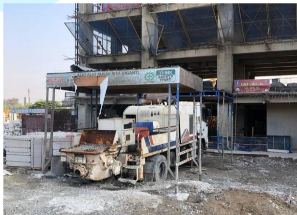
Gambar 3. 14 Lokasi Concrete Pump
