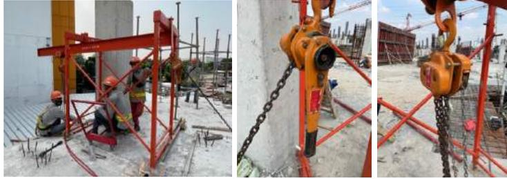
**Gambar 3.18 Stressing Frame, Chain Block, dan Level Block**
