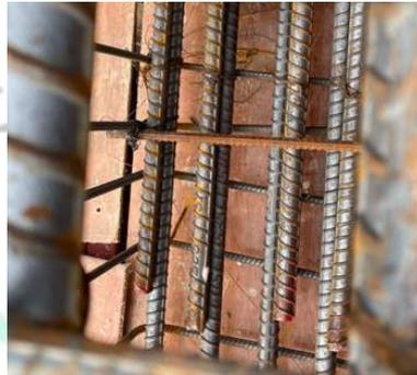
**Gambar 3.42 Support Bart Installation**
