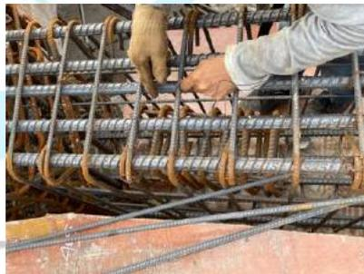
**Gambar 3.43 Install Bursting Link**
