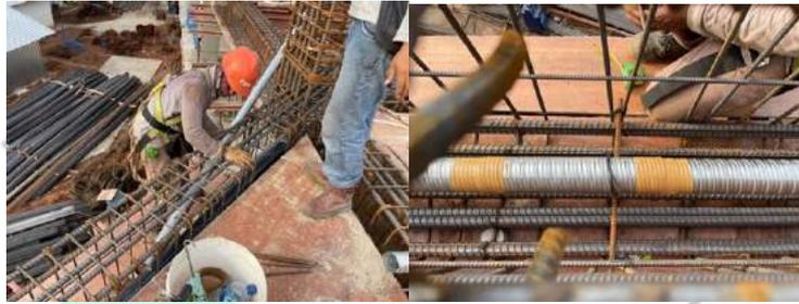
**Gambar 3.44 Duct Installation**
