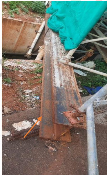
Gambar 3. 22 Kaki Shoring beam WF 300 x 300
