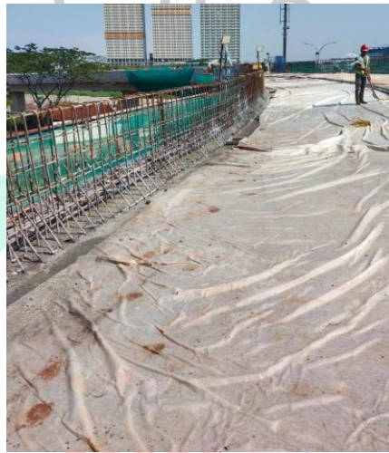
Gambar 3. 38 Proses Perawatan Beton
