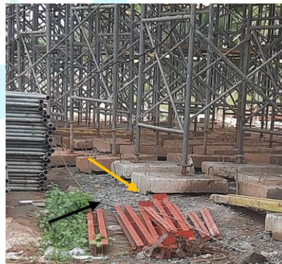
Gambar 3. 14 Steel Waller U100 SRGZ
