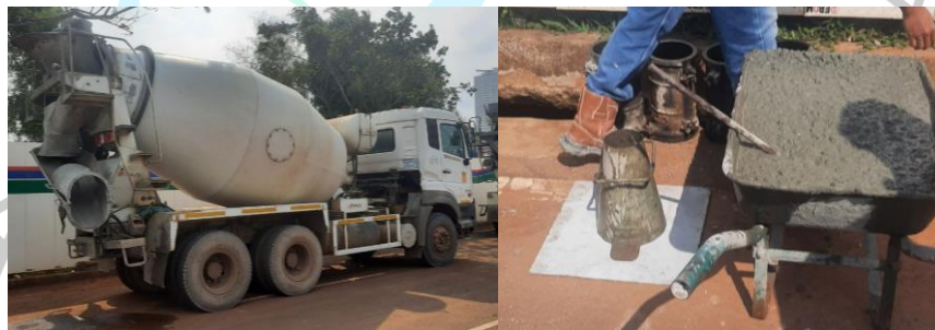
Gambar 3. 8 Beton Ready Mix
