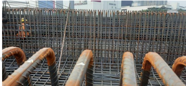
Gambar 3. 25 Instalasi Besi Dinding Box girder
