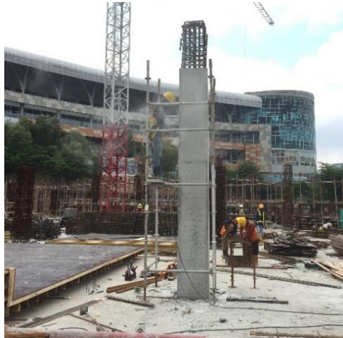
Gambar 3.20 Proses Grouting Kolom
