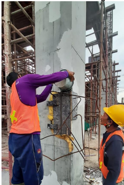
Gambar 3.20 Proses Grouting Kolom
