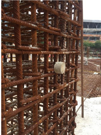
Gambar 3.4 Beton Decking
