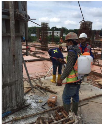
Gambar 3.19 Proses Curing Kolom
