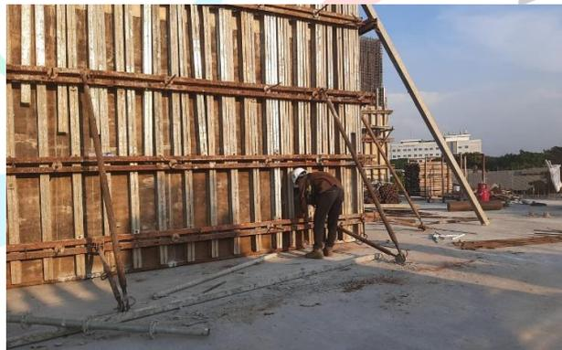
**Gambar 3. 31** *Verticality Test*
