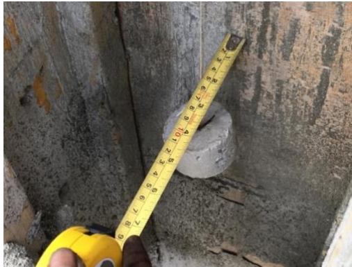
Gambar 0.50 Verticality Test di Core Wall
