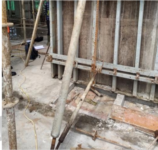
Gambar 0.48 Bracket Push Pull Dipasang di Bekisting Core Wall
