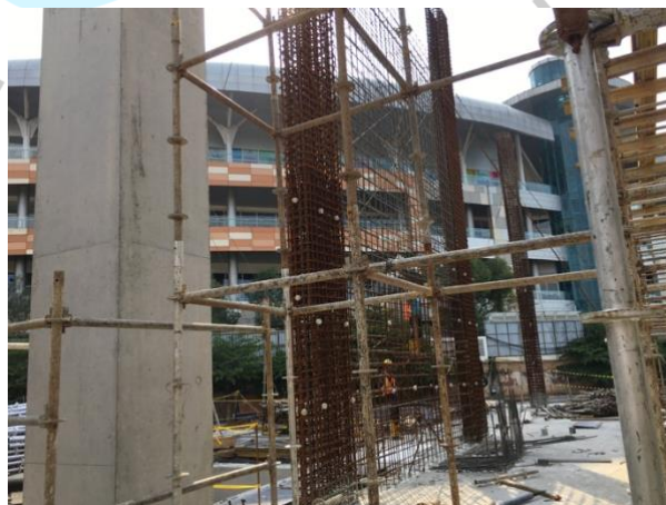
Gambar 0.27 Beton Decking Terpasang di Shear Wall
