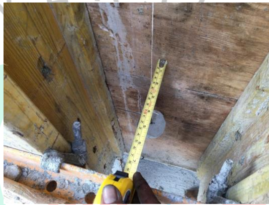
Gambar 0.35 Verticality Test di Shear Wall
