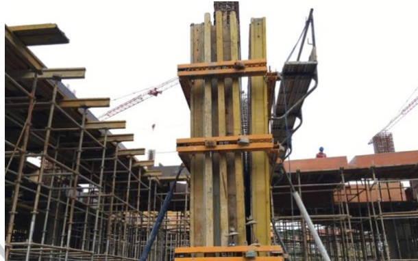
Gambar 0.51 Proses Pelepasan Bekisting Core Wall
