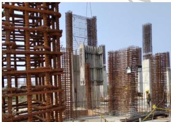
Gambar 0.38 Proses Pelepasan Bekisting Shear Wall
