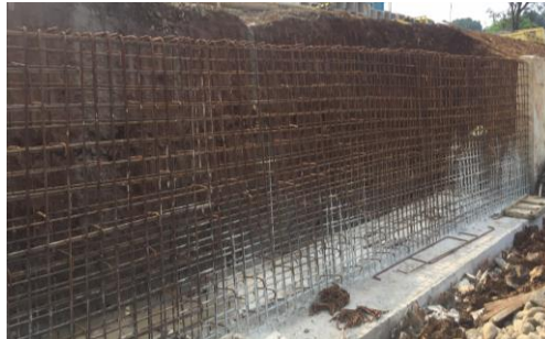
Gambar 3.23 Pembesian Body Retaining Wall (Sumber : Data Pribadi)
