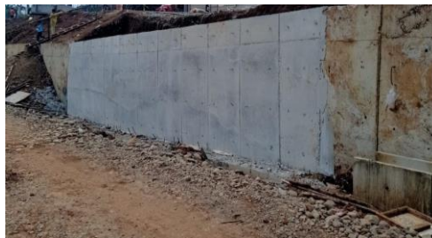
Gambar 3.25 Finishing Body Retaining Wall (Sumber : Data Pribadi)
