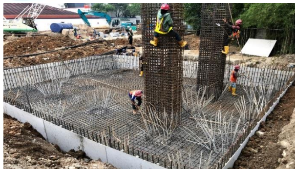
Gambar 3. 49 Instalasi Besi Pile Cap
