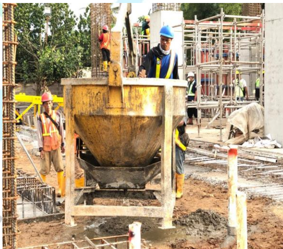
Gambar 3. 22 Concrete Bucket
