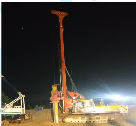
Gambar 3. 26 Hydraulic Boring Crane
