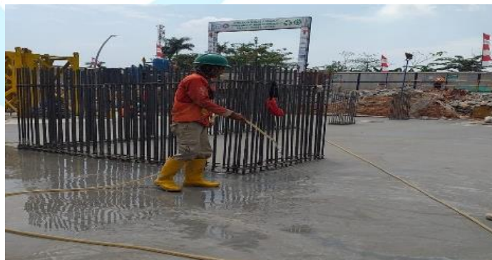
Gambar 3. 51 Proses Curing Beton
