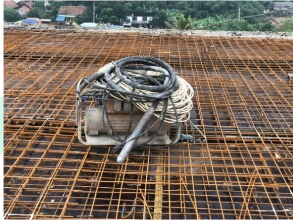
Gambar 3. 23 Concrete Vibrator
