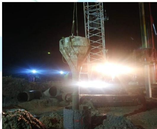
Gambar 3. 36 Concrete Bucket
