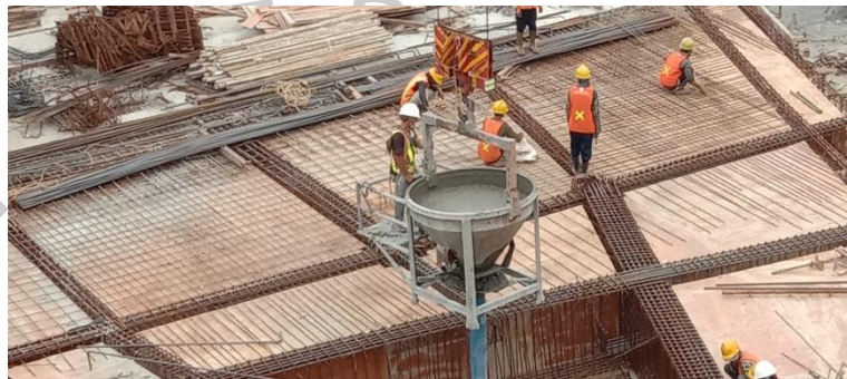
Gambar 3. 18 Concrete Bucket
