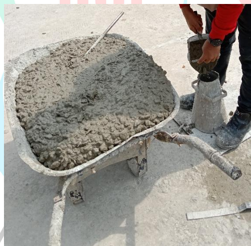
Gambar 3. 14 Beton Ready Mix
