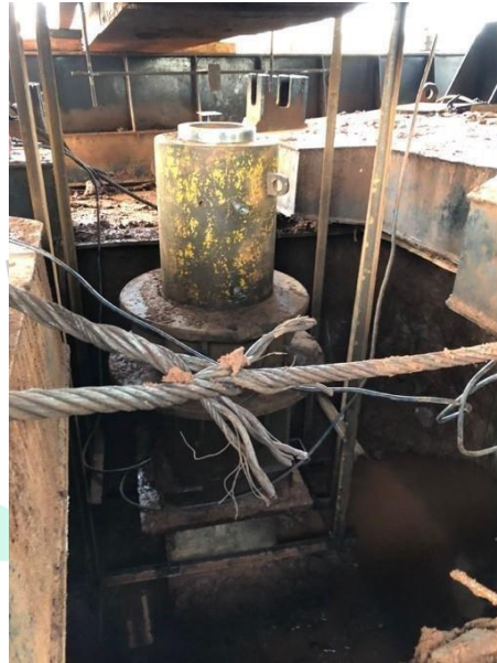
Gambar 3. 21 Persiapan Loading Test
