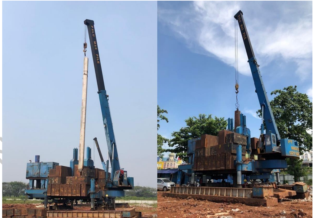
Gambar 3. 8 Alat Kerja Hidraulic Static Pile Driver (HSPD)
