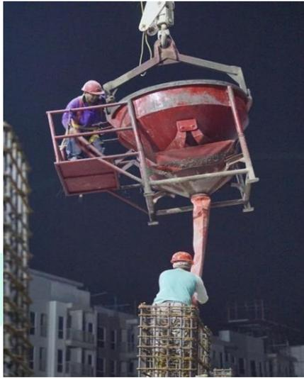
**Gambar 3. 43 Concrete Bucket**
