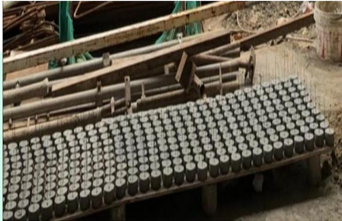
Gambar 3. 55 Beton *Decking*
