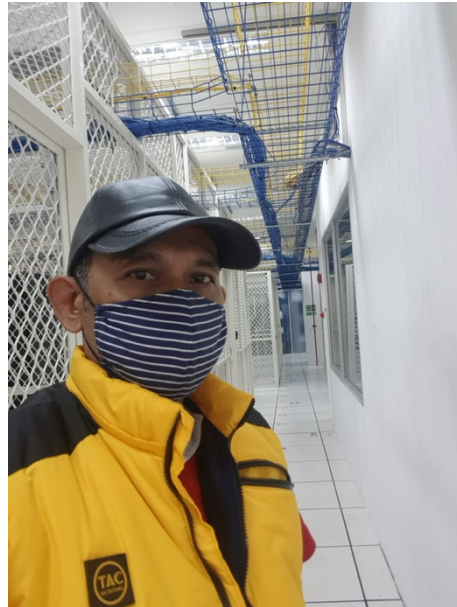
Gambar 1.2. Ruang Data Center
