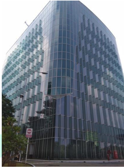
Gambar 1. 1 Beltway Office Park Tower B Sumber : Dokumentasi Praktikan, 2021
