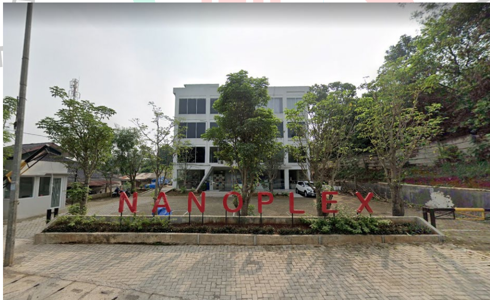
Gambar 1.2. Gedung Kantor PT.Graha Nano Tech Indonesia
