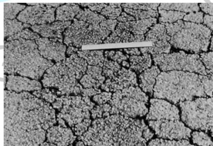
Gambar 2.1 Retak Kulit Buaya (*Alligator Cracking*) (ASTM D 6433 – 07)
