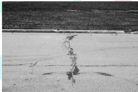
Gambar 2.5 Retak Sambungan Pelebaran Jalan (Widening Cracks) (ASTM D 6433 – 07)
