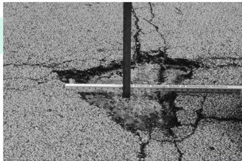
Gambar 2.13 Lubang (*Potholes*) (ASTM D 6433 – 07)
