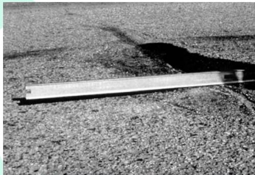
Gambar 2.11 Jembul (*Upheaval*) (ASTM D 6433 – 07)
