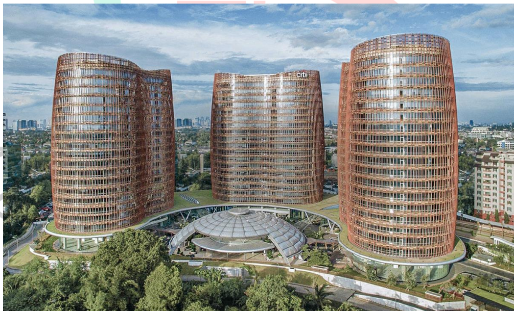
Gambar 1.1 Gedung South Quarter
