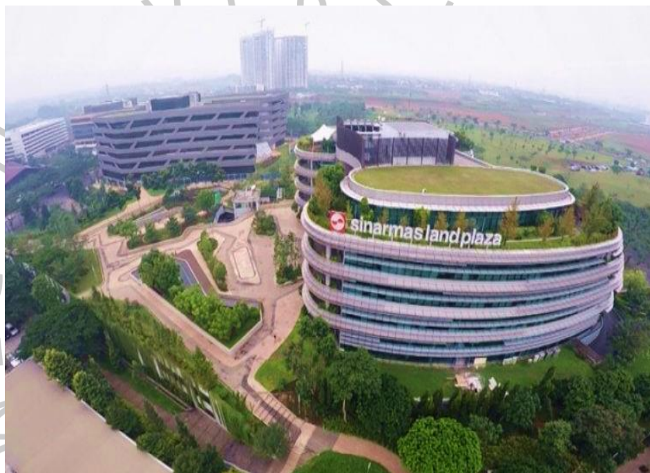
Gambar 2. 2 Gedung Sinar Mas Land Plaza BSD City
