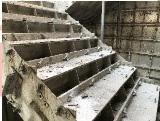
Gambar 3.57 Setting Bekisting Tangga
