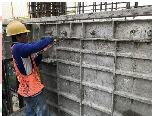
Gambar 3.55 Setting Bekisting Vertikal
