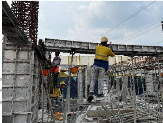
Gambar 3.56 Setting Bekisting Balok
