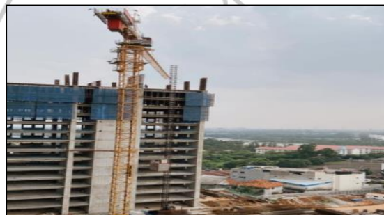
Gambar 3.7 Tower Crane Proyek Kingland Avenue
