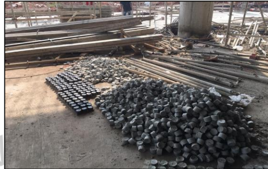
Gambar 3.6 Beton Decking
