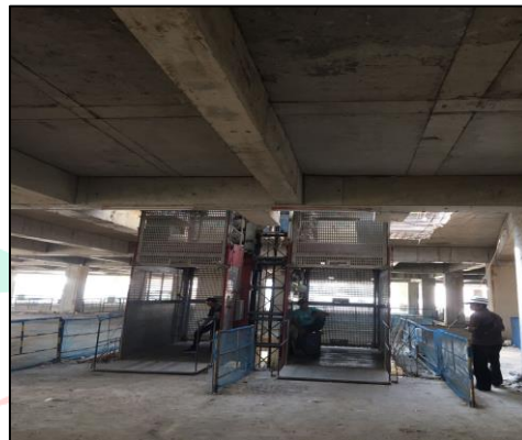
Gambar 3.14 Passenger Hoist
