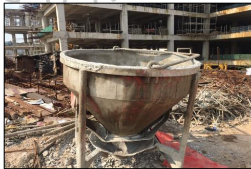
Gambar 3.13 Concrete Bucket
