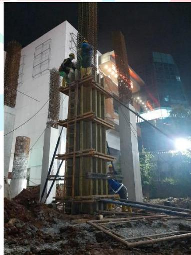
Gambar 3. 11 Bekisting Kolom.
