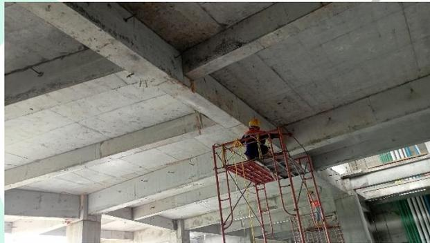
Gambar 3. 26 Proses Gerinda Repair Balok.
