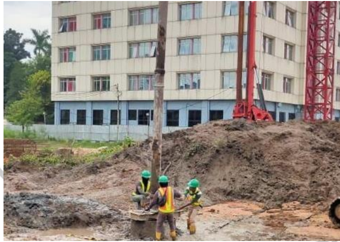
Gambar 3. 30 Instalasi Pipa Tremie
