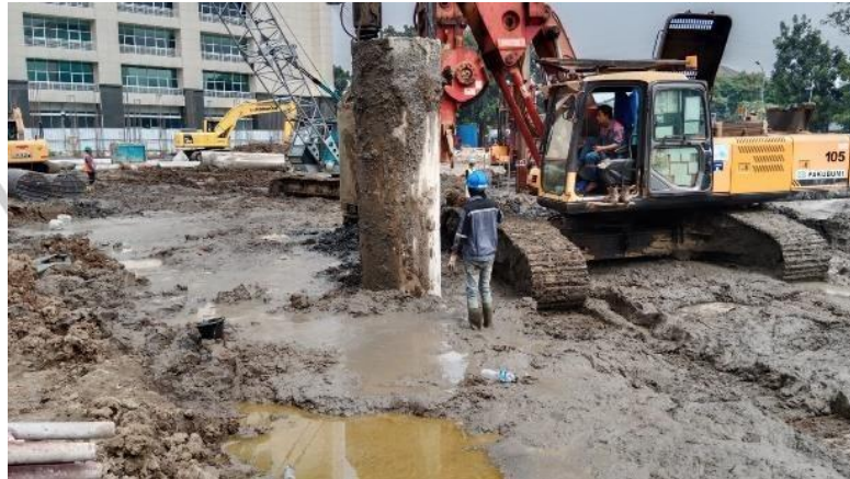
Gambar 3. 23 Pemasangan temporary casing
