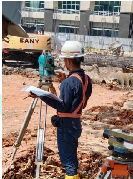
Gambar 3. 11 Penentuan titik bored pile
