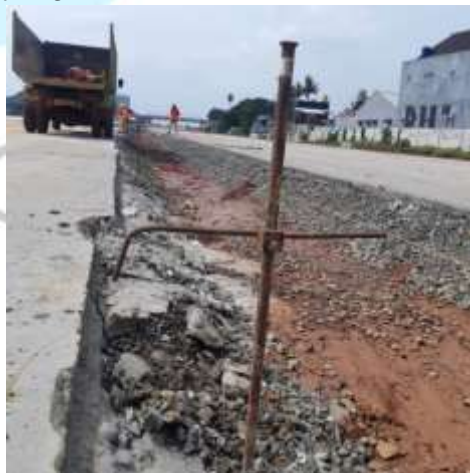
Gambar 3.9 Marking Patok
