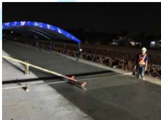
Gambar 3.46 Proses Grooving
