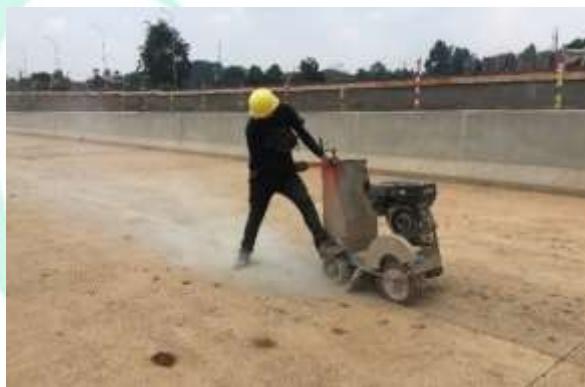
Gambar 3.47 Proses Cutting
