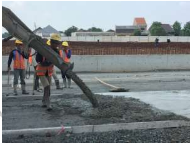
Gambar 3.37 Proses Pengecoran Lean Concrete
