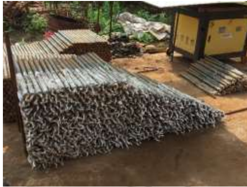
Gambar 3.24 Dowel Bar
