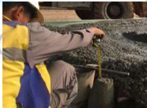
Gambar 3.40 Uji Slump Rigid Pavement
