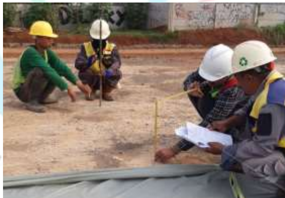
Gambar 3.38 Proses Laveling Rigid Pavement
