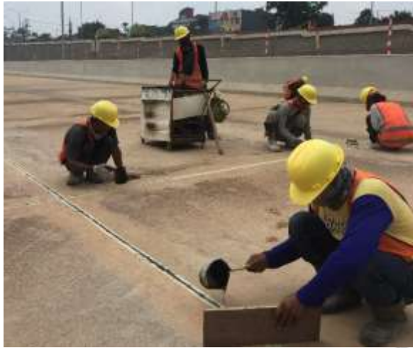
Gambar 3.48 Proses Joint Sealent
