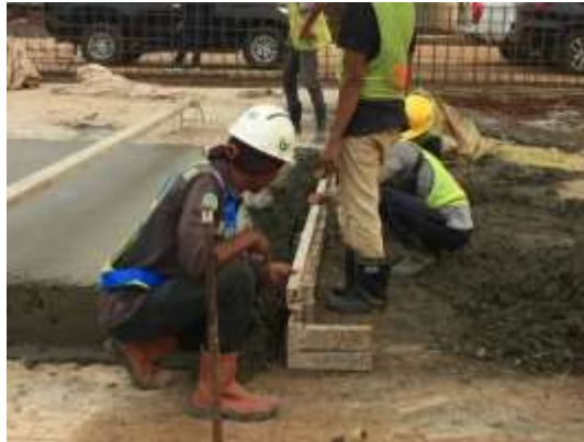
Gambar 3. 45 Proses Pemasangan Stoper Chair
