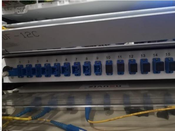
**Gambar 3.14 Optical Termination Box (OTB)**
