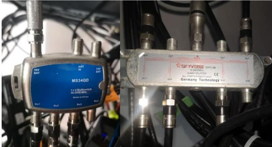
Gambar 3.12 Splitter coaxial
