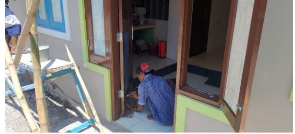
© pekerjaan pengecatan kusen
