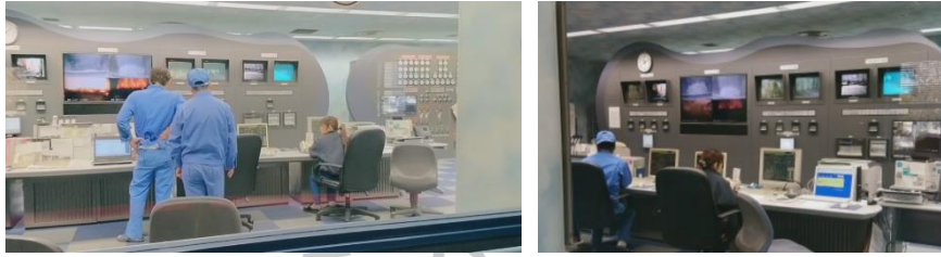
Gambar 2. 17 Ruang Kontrol Panel Maishima Sumber: https://youtu.be/FDNcahZcG_Y , 2022
