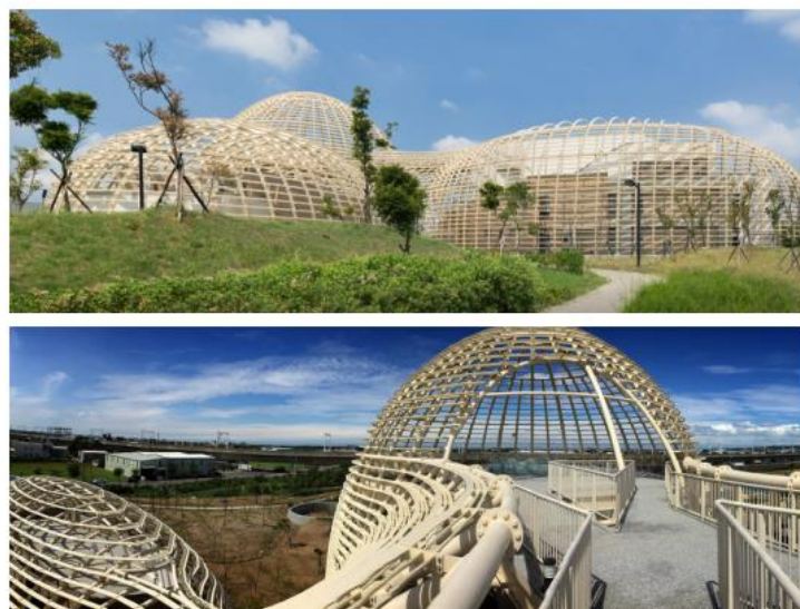
Gambar 2. 3 Fasad Touyan Sawage Treatment Sumber: Archdaily, 2017
