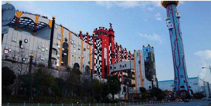
Gambar 2. 7 Fasad Maishima Incineration Plant Sumber: https://youtu.be/FDNcahZcG_Y , 2022
