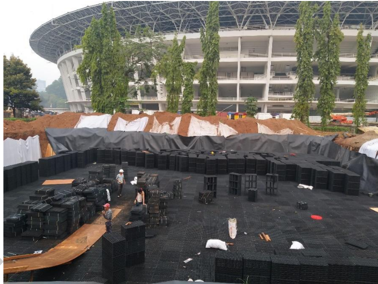
Gambar 2.10 Proyek Prasarana Gelora Bung Karno (Magnatank.com, 2023)
