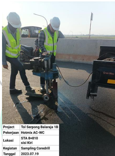
Gambar 2. 9 Sampling Coredrill Asphalt jembatan mainroad (Source : Dokumentasi pribadi)
