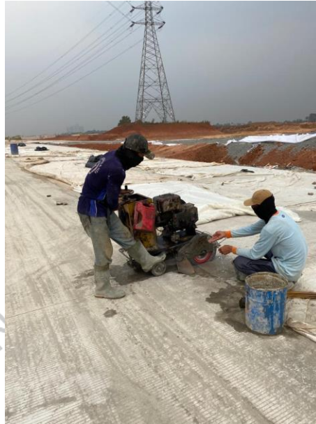
Gambar 3. 25 Proses Cutting rigid pavement (Source : Dokumentasi pribadi)
