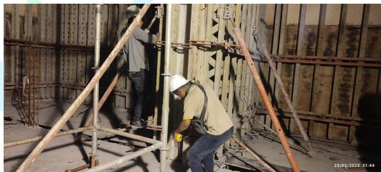
**Gambar 3. 54 Proses Pelepasan Bekisting Dinding Geser**
