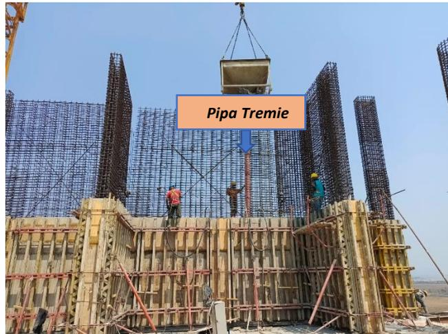
**Gambar 3. 51 Pengecoran Dinding Geser**
