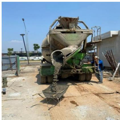
**Gambar 3. 8 Beton Ready Mix**
