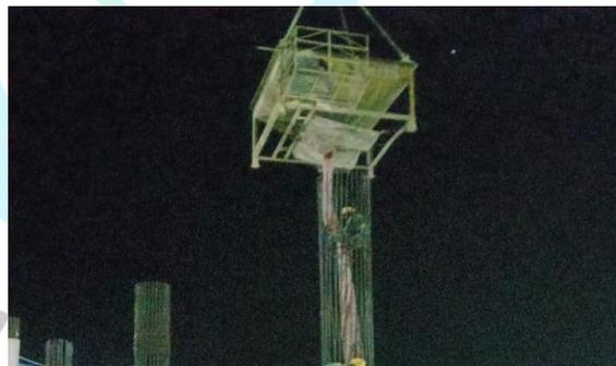
**Gambar 3. 22 Concrete Bucket**
