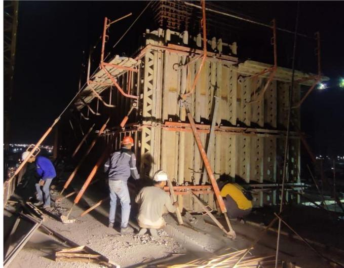
**Gambar 3. 46 Proses Pengecekan Verticality Bekisting Dinding Geser**
