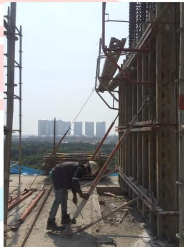
**Gambar 3. 43 Pemasangan Bracket Push Pull Bekisting Dinding Geser**
