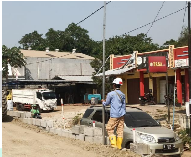
Gambar 3.12 Marking Patok
