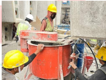
Gambar 3. 46 Grouting
