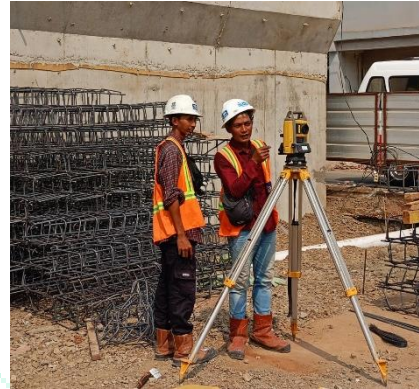
Gambar 3. 31 Stacking Out
