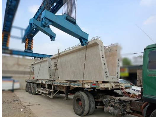
Gambar 3. 30 Precast Girder PC U
