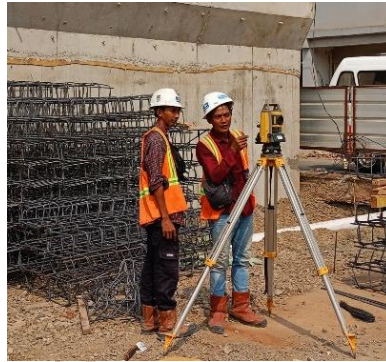
Gambar 3. 39 Stacking Out
