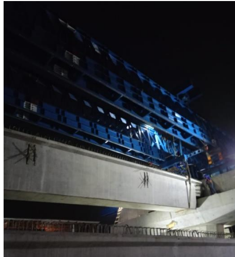
Gambar 3. 47 Erection Girder
