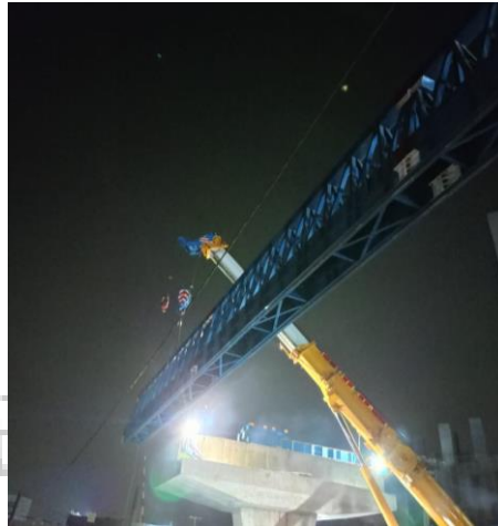
Gambar 3. 41 Instalasi Launcher
