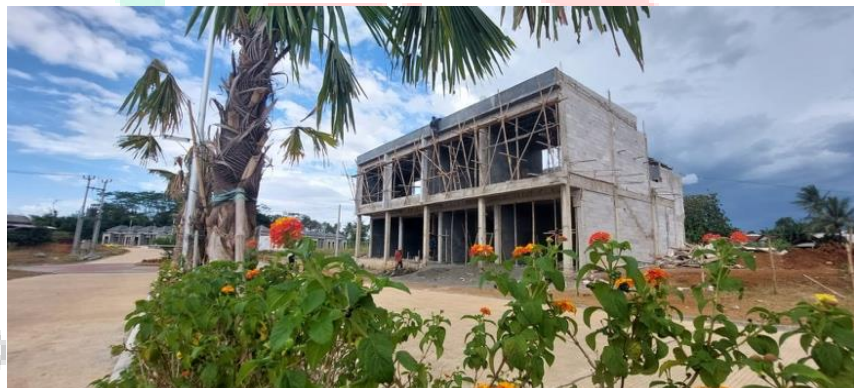
Gambar 2. 8 Proyek Perumahan Tropical Village (Sumber: Dokumentasi Pribadi)
