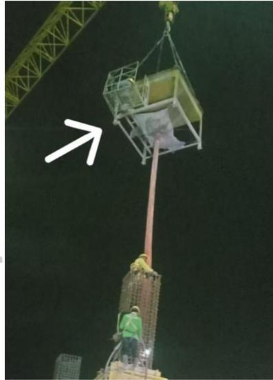
Gambar 3. 16 Concrete Bucket
