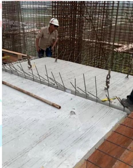
Gambar 3. 28 Pemasangan *Half Slab Precast*
