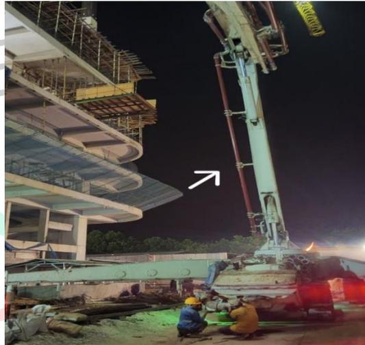
Gambar 3. 18 Concrete Pump
