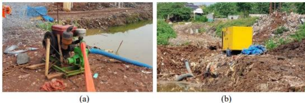
Gambar 3. 16 Alat dewatering: (a) small water pump generator; (b) big water pump generator
