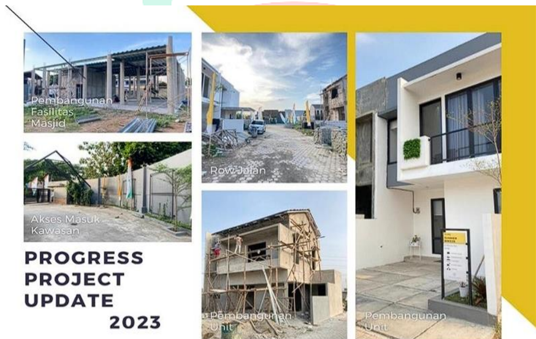
Gambar 2. 5 Proyek Grand Al Ihsan Premiere Sumber : PT. Nuraria Properti Indonesia
