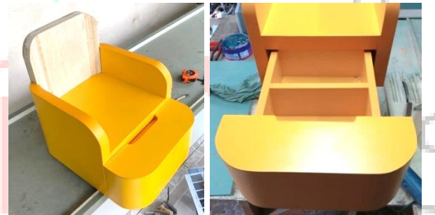
Gambar 4. 16 pemasangan HPL ((High Pressure Laminate)
